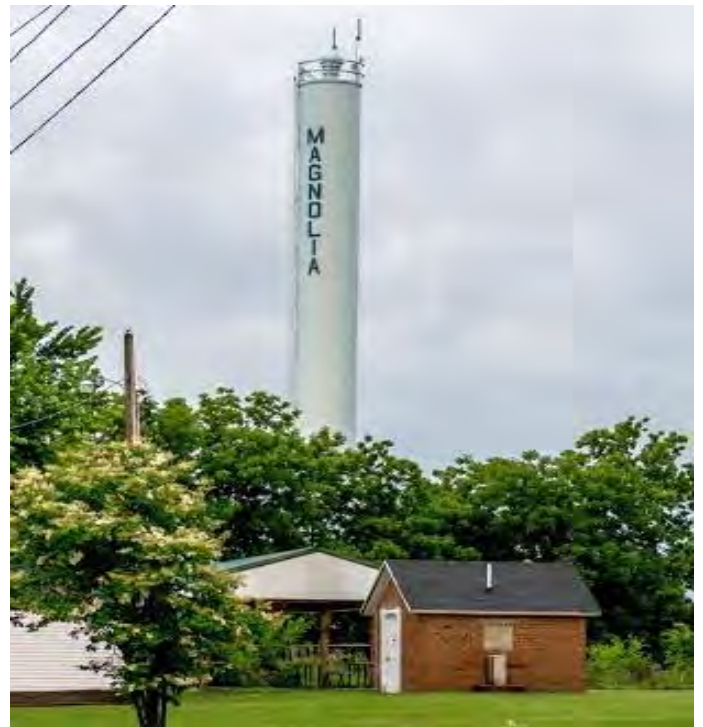
The Village of Magnolia, IL and their new 53,000 Gallon Water Tower
